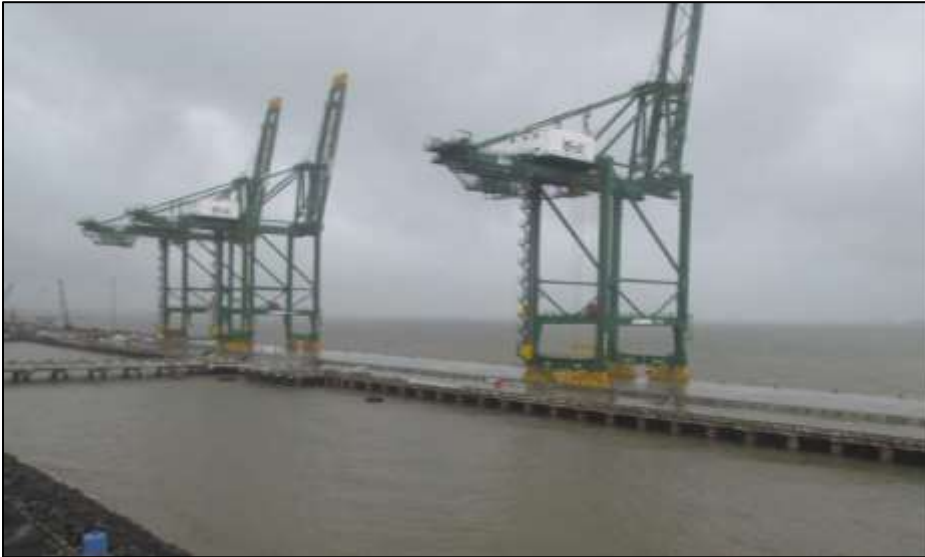
Caption – BMCT is nearing completion
